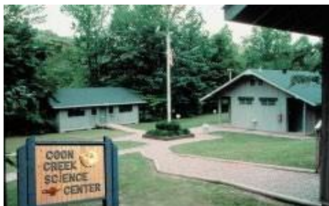
Figure 4. Coon Creek Science Center facilities
